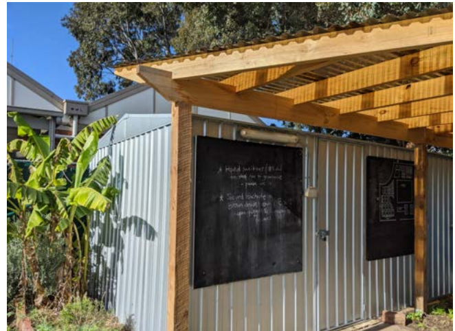
Photo 5: The shed and adjacent verandah were upgraded in March 2020
